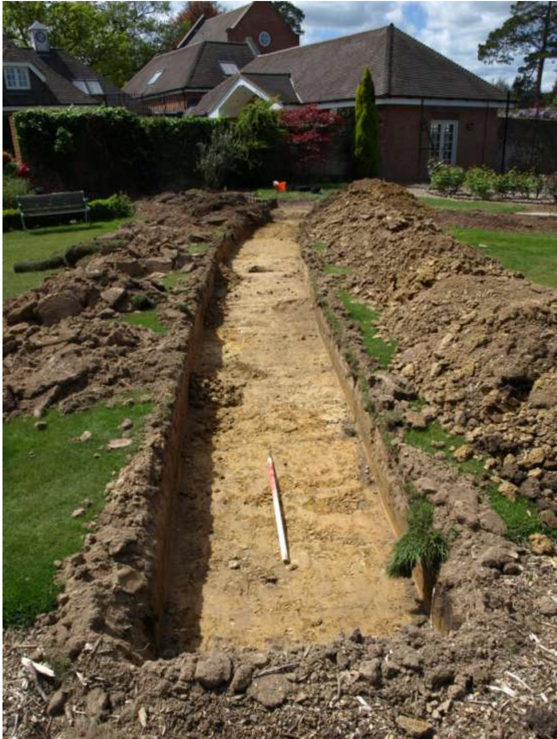
Plate 5. Trench 1 looking west (1m scale)
